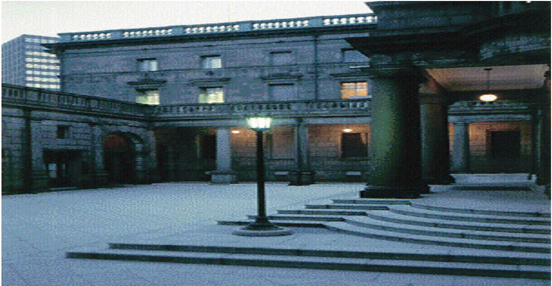
View of the BOJ courtyard around sunset
